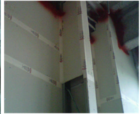
The double wrapped corner
