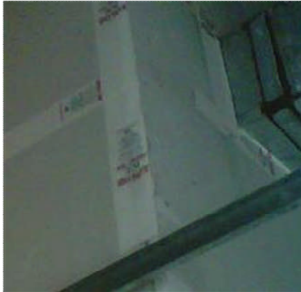
Proper wrapped corner
